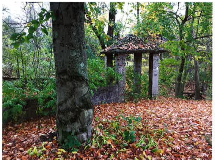
Small stone gazebo built by Jac. Donges where walkers could start their ravine hikes
